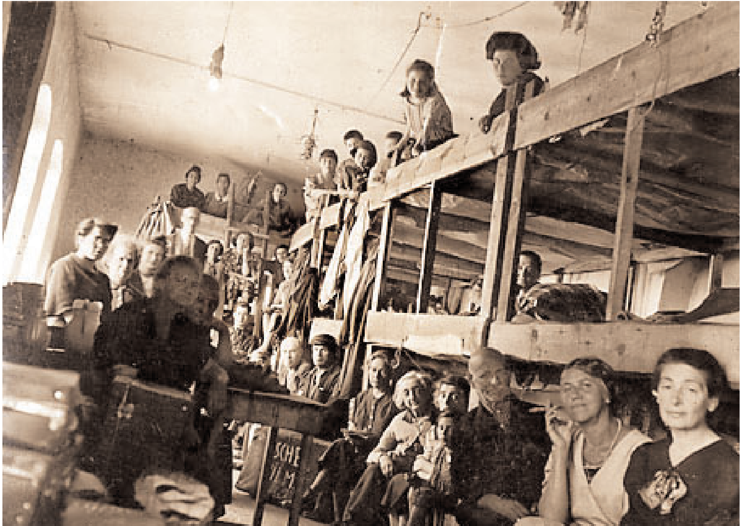
This is a picture of one of the mass accommodations in Opole ghetto, Poland, which my father had taken by a local Jewish photographer in May 1941. My parents, Wilhem and Johanna Schischa [nee Friedmann], were deported to Opole ghetto in Poland from Vienna on 26th February 1941. They were murdered a year later in either Belzec or Sobibor concentration camp.
